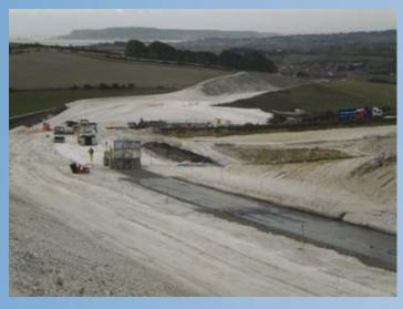
foundation. This would enable a road construction of just 250mm of blacktop to be laid directly onto the stabilised chalk. This process was successfully pioneered by McArdle Stabilisation on the Polegate Bypass and A6 Higham Ferrers to Rushden Bypass. The process has been adopted by the Specification for Highways Works as an approved construction method and is now becoming more widely used across the UK.
